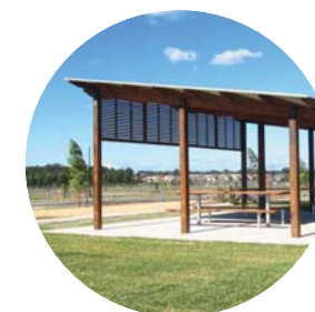
Picnic Shelter (Image: Landmarkpro)
