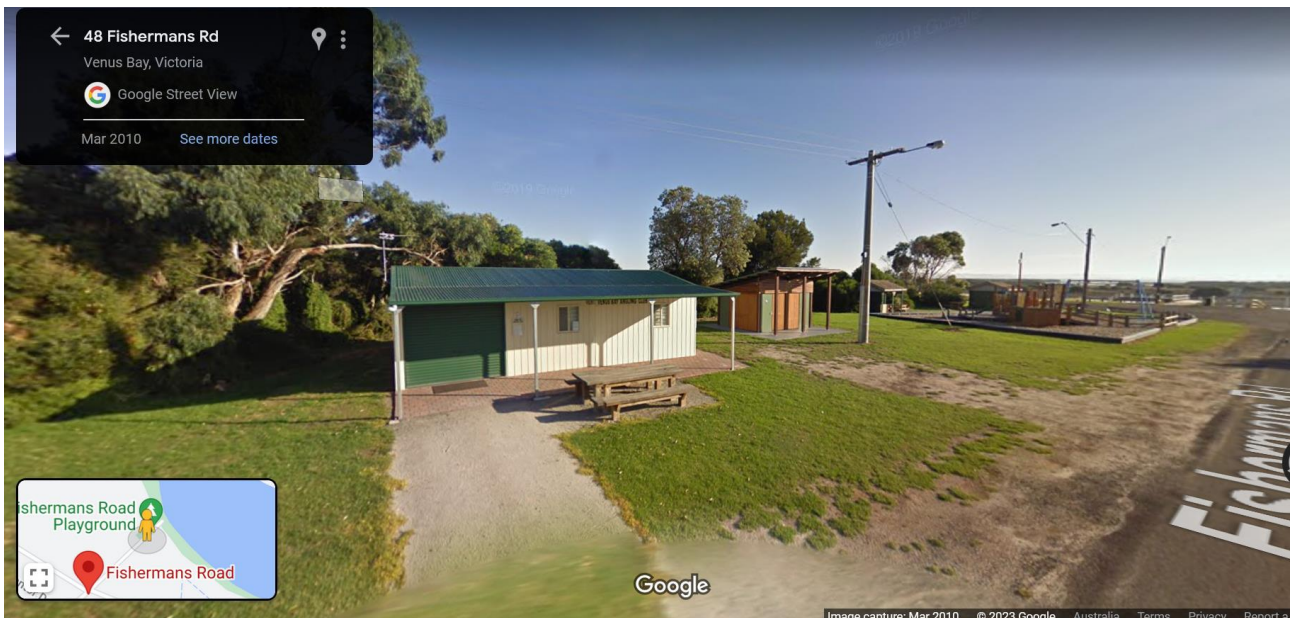
Figure 13 Fishing club, playground, jetty and three phase electricity supply
